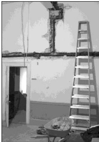
Installing the sprinkler system
