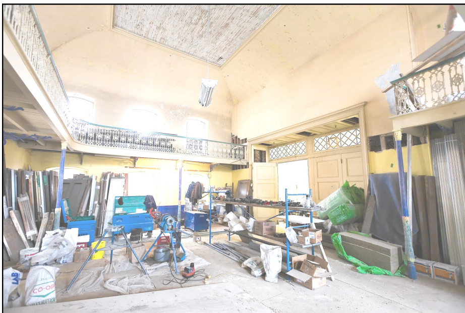
The College Hall under restoration in 2006 (Photo Paul Dionne)
