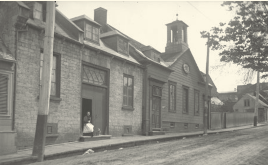
Jeffery Hale's Sunday School on St. Joachim Street in 1906, now demolished (on the right of this photo, with steeple) BAnQ
