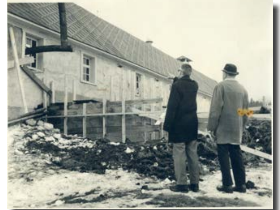
Construction site of the Piggery Theatre, Piggery Theatre fonds P001/004/001
