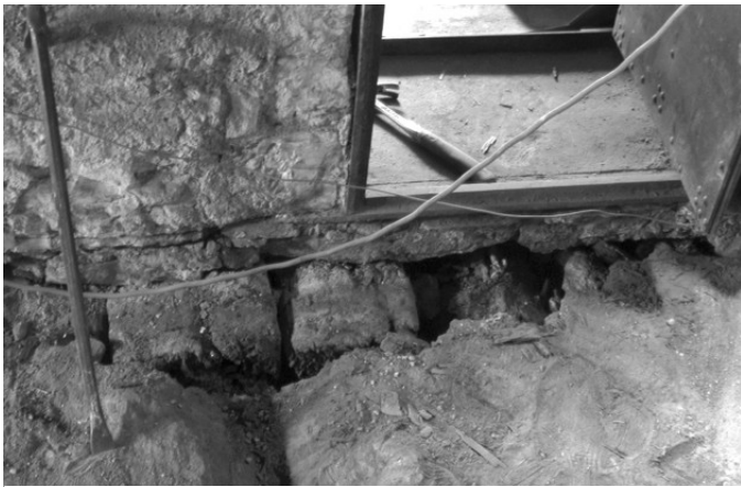
Fig. 6: Wooden beams under the walls
