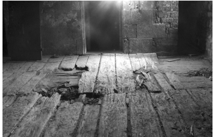
Fig. 1: The French tradition of laying planks
