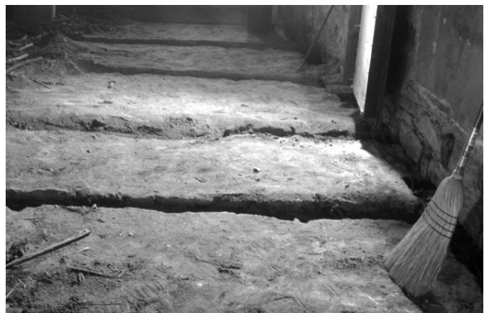
Fig. 4: Mortar sub-floor with troughs for the pine joists
