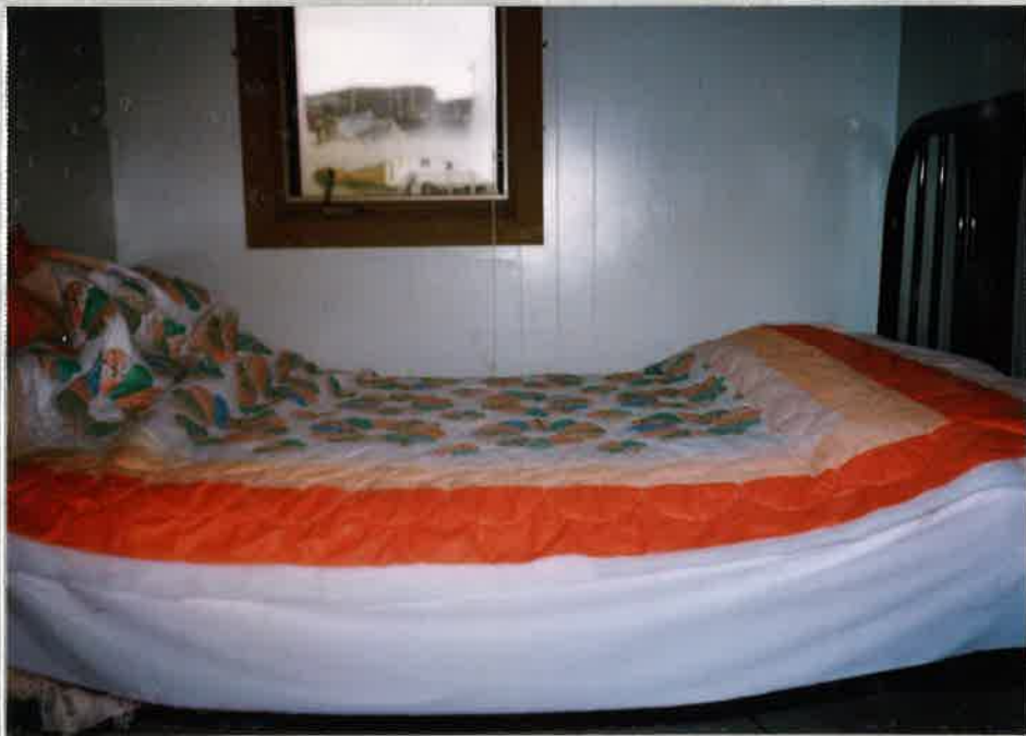
White lining not completed
